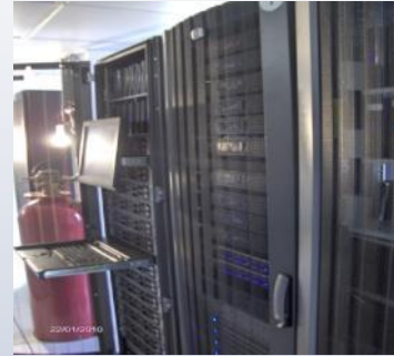
Rack assembly and hardware installation
