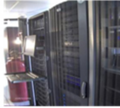
Rack assembly and hardware installation
